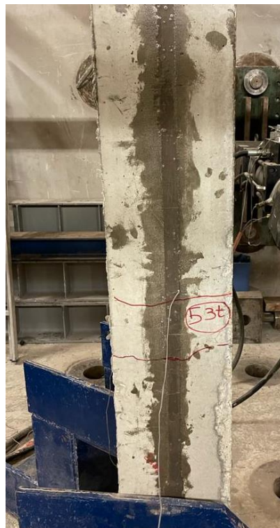
Figure 4.6 Cracks at the tension side of Column 1.5-C08-2
