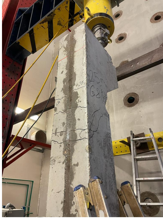
Figure 4.41 Cracks at the tension side of Column 2.5-C08-1
