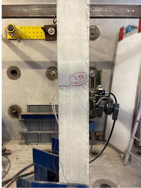
Figure 4.17 Cracks at the tension side of Column 2-C00-1
