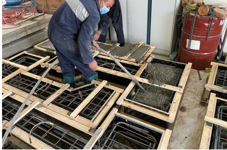
Figure 3.13 Casting the concrete
