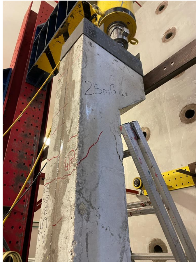
Figure 4.47 Cracks at the tension side of Column 2.5-C12
