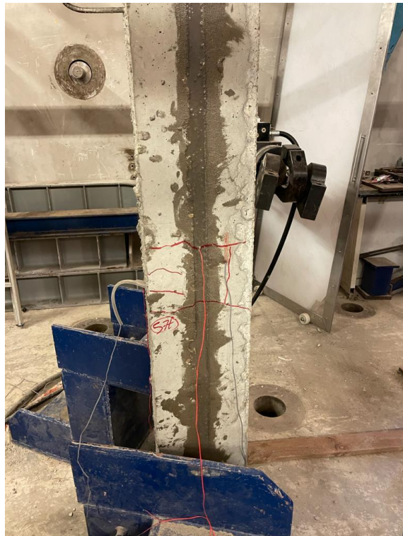
Figure 4.12 Cracks at the tension side of Column 1.5-C12-2
