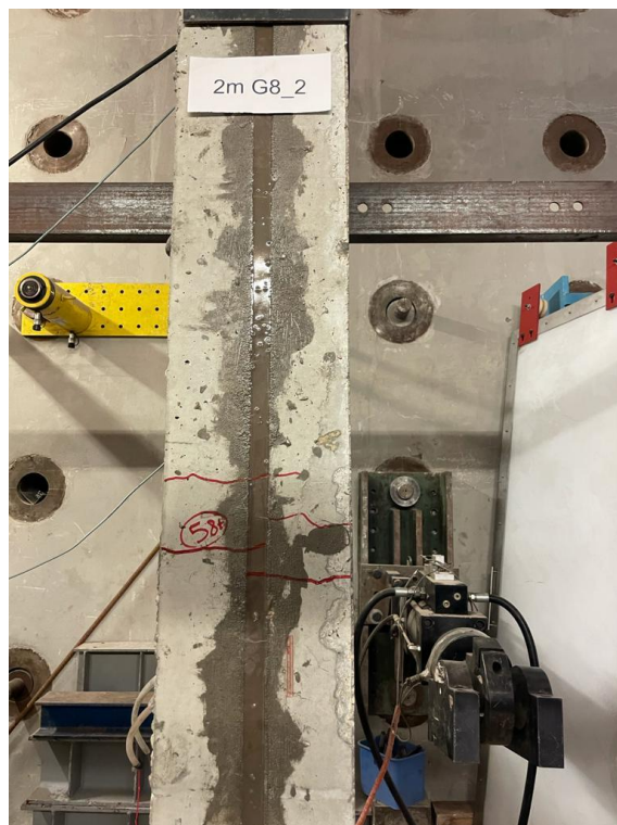
Figure 4.24 Cracks at the tension side of Column 2-C08-2
