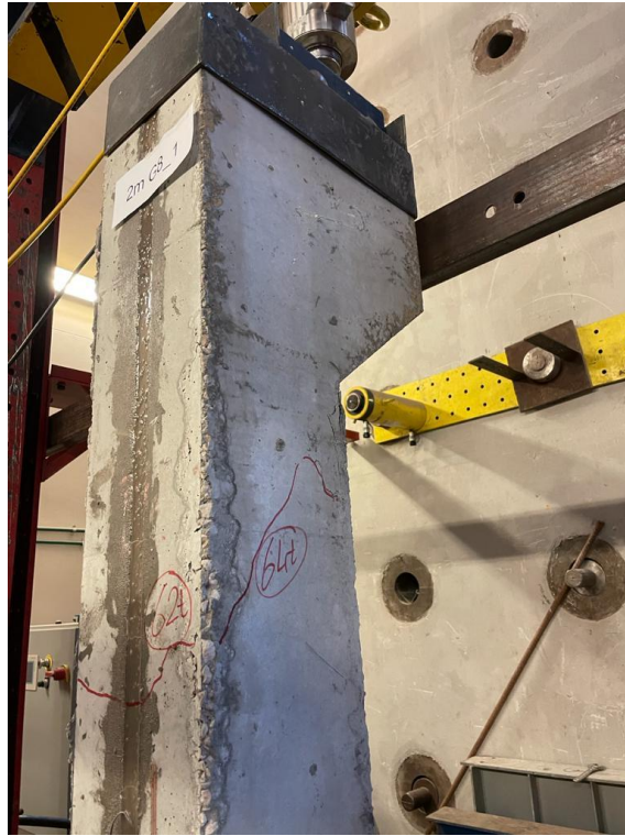
Figure 4.23 Cracks at the tension side of Column 2-C08-1
