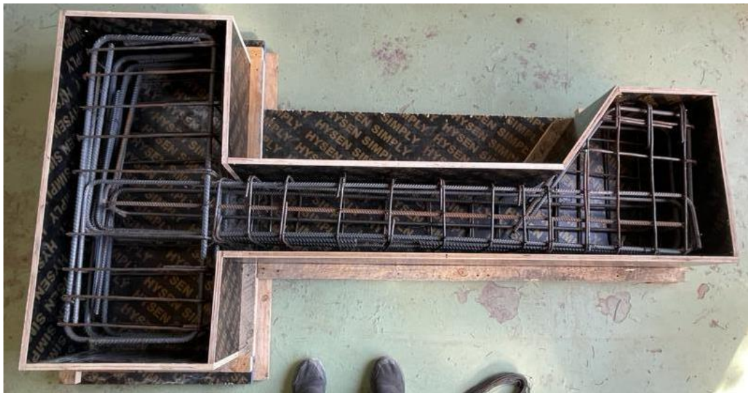
Figure 3.10 Steel reinforcement placed in the formwork
